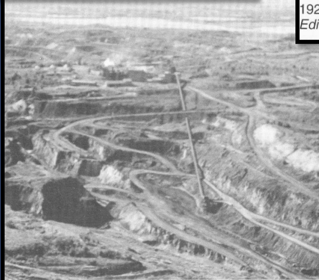
The Portsmouth Pit on the Cuyuna Range in North Crosby.
