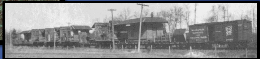
The Soo Line depot was cut into sections for the move to Riverton.
